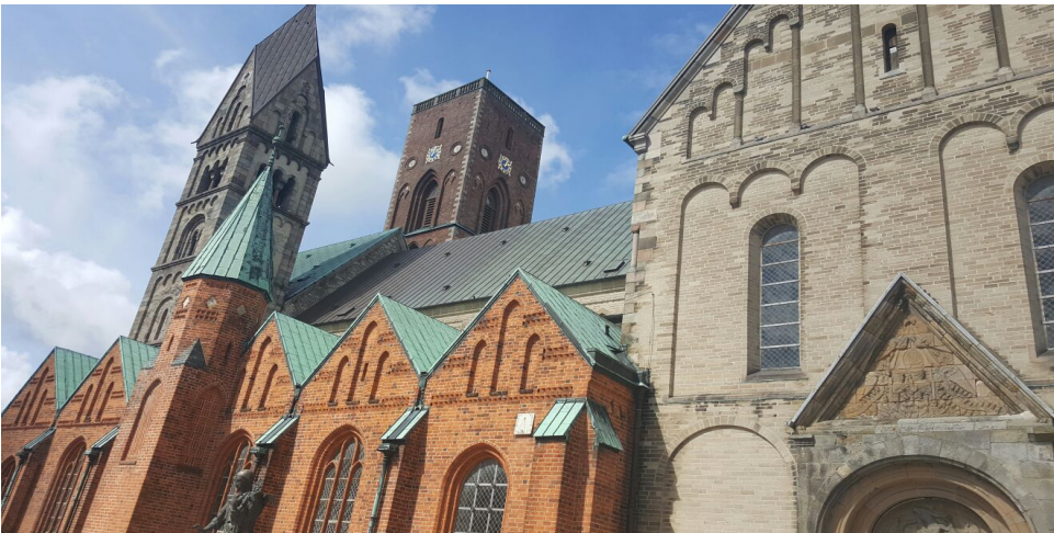
The side of Ribe's main cathedral, the lighter part was the original church while the bricks were added later after an earthquake and the consequential risk of collapse.
